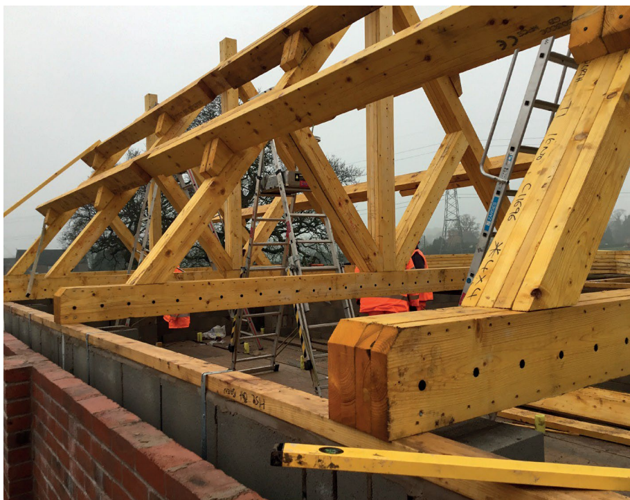
Drayton Basset Timber Roof Construction
