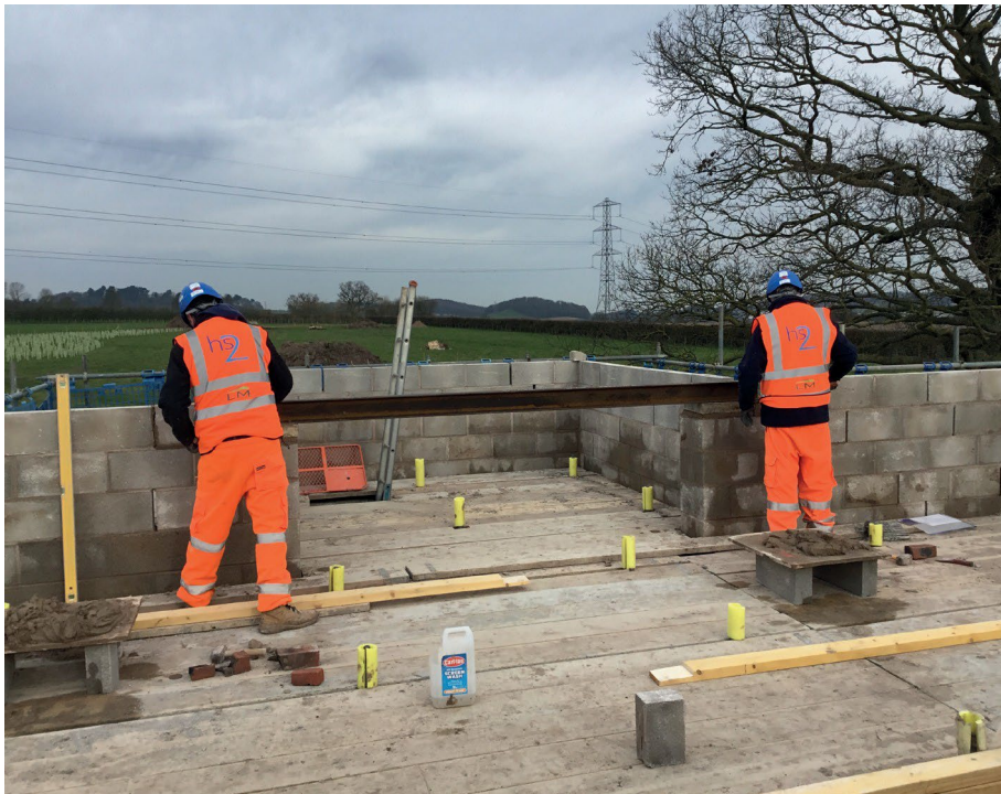
Installation of Steel Beam - Drayton Basset Bat Barn
