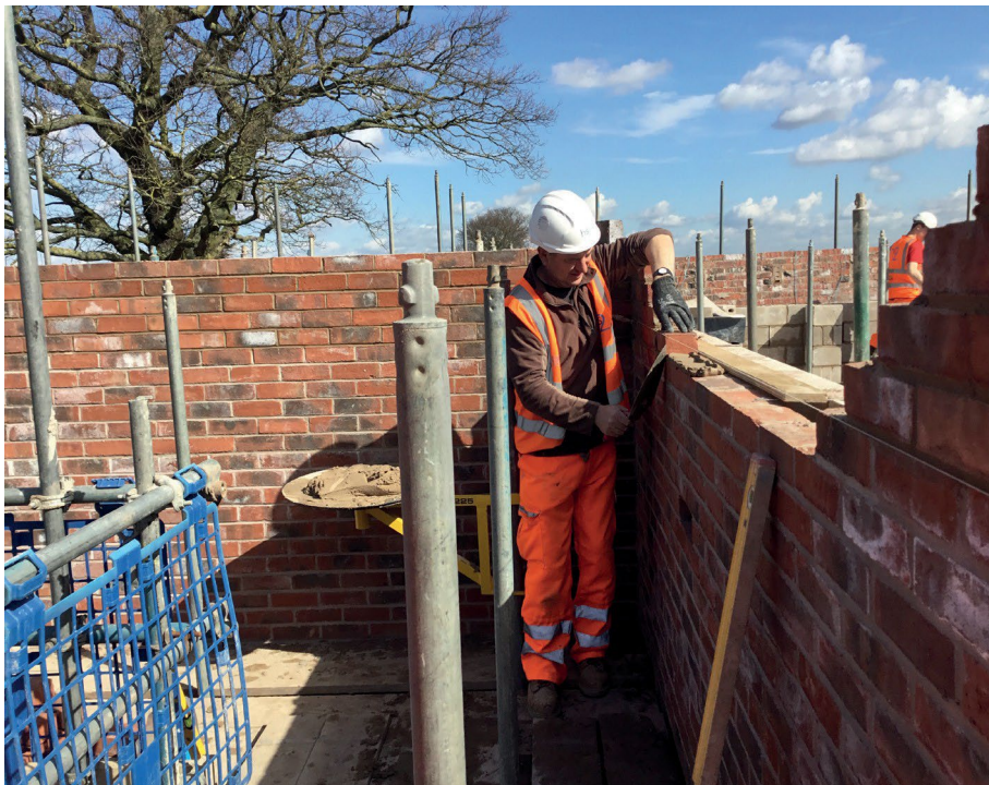
Brick Work on Drayton Basset Bat Barn
