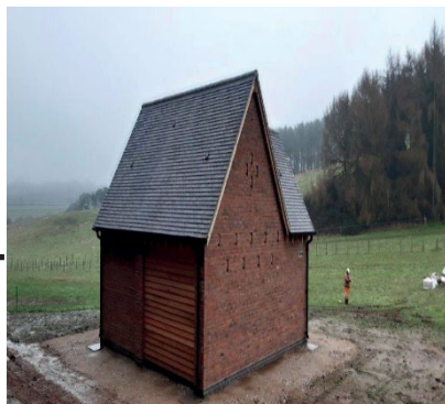
Hints - Completed Bat Barn
