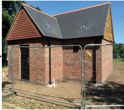
Curdworth - Completed Bat Barn
