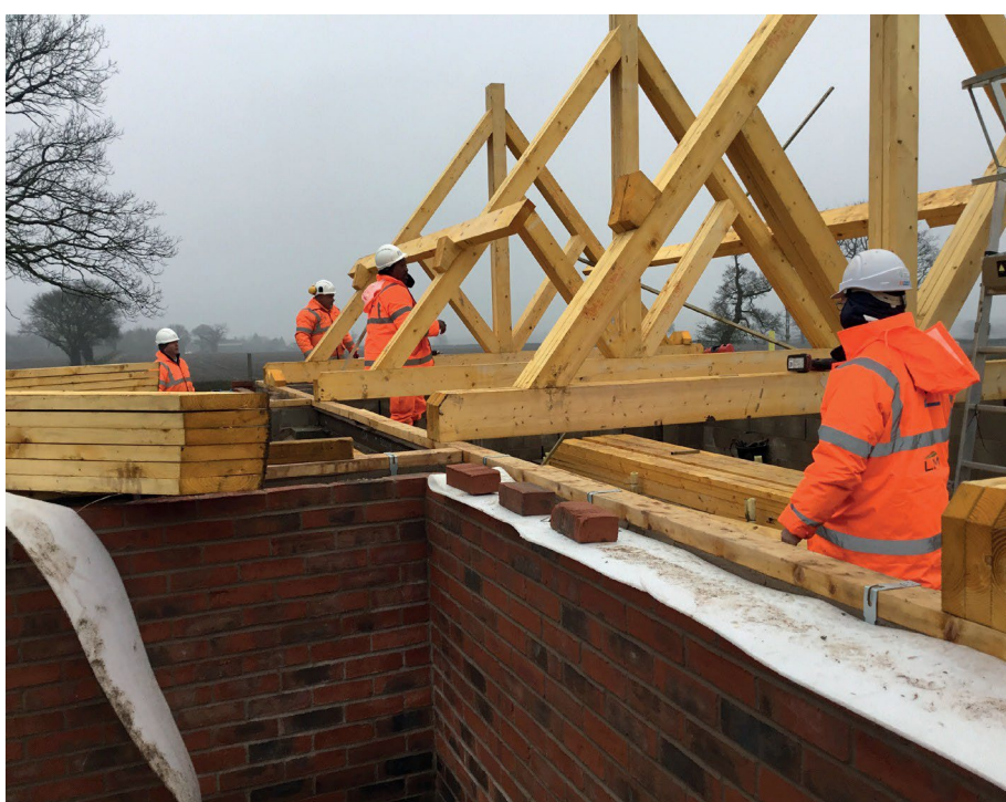
Drayton Basset Timber Roof Construction
