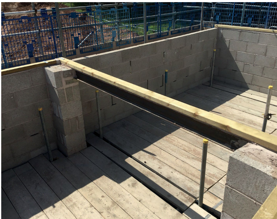
Installation of Steel Beam - Hints Bat Barn
